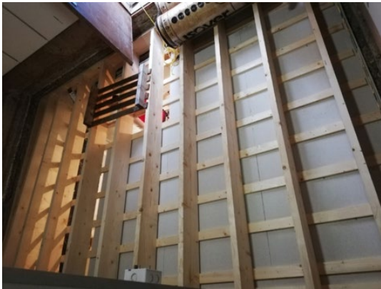
Figure 2. Installation of the bare timber frame floor in the test stand.
