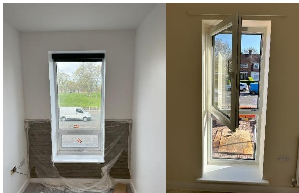
Photo 1: Site 1 Window Photo 2: Site 2 Window Open
