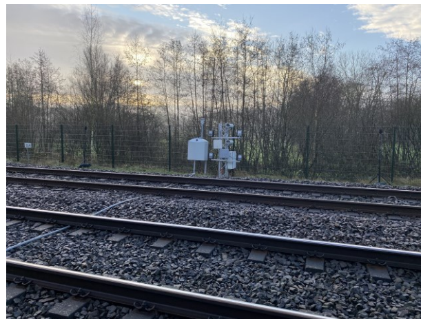
Figure 2. Onsite installation of one of the two N-RSD systems for NEMO.
